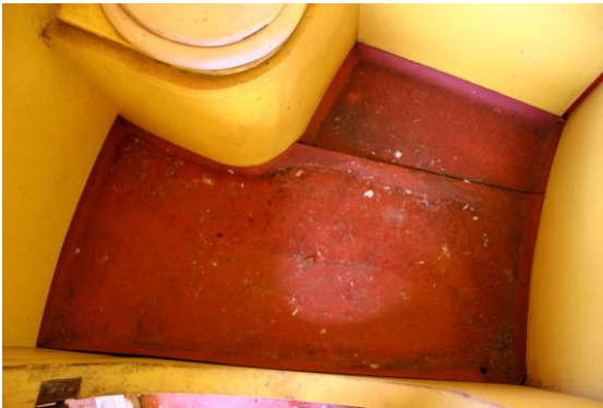
Figure 63. The floor of the toilet.
