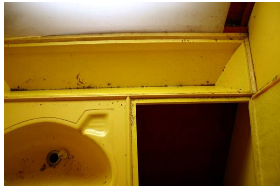
Figure 62. Uplifted table top decks.
