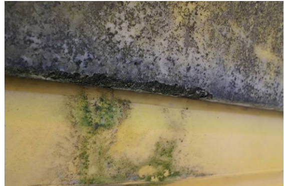
Figure 93. The edge of the small shelter has worn away. Some micro-organism was detected.
