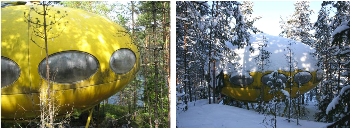
Figure 100. (left) A photograph taken in September 2009 shows the roof condition. Figure 101. (right) Snow covers the roof.
