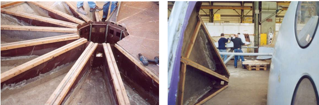
Figure 41. The floor plates are partially dismantled. (Rasier 2002)
